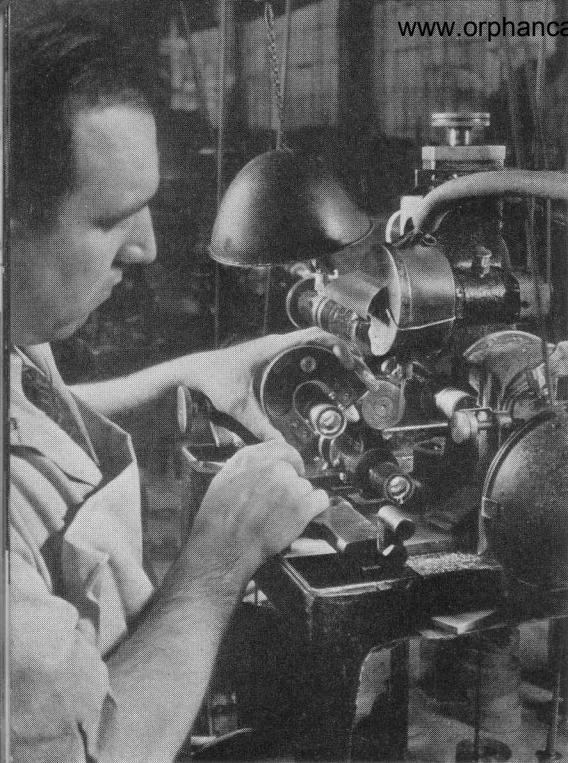
● Centering and edging—Each lens element must be centered accurately and its edge ground to fit the mount.
